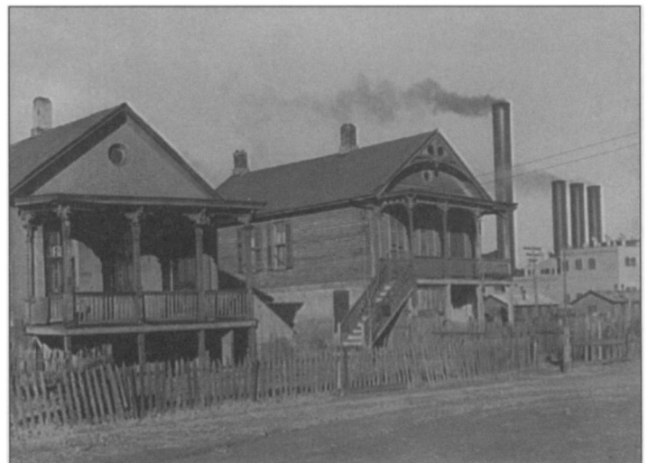
Houses near the Nebraska Power Company Plant. Omaha, Nebraska, November 1938. Photograph by John Vachon. (Courtesy of the Library of Congress, LC-USF34-T01-008878-D.)
